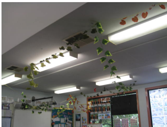
Photograph 3: Lights on in empty rooms
