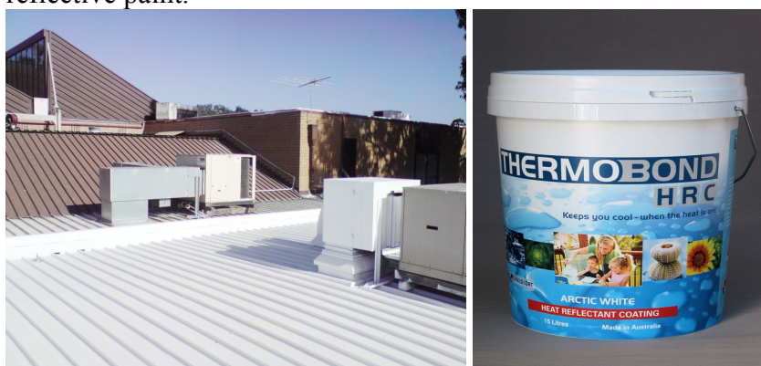
Photograph 17: Heat reflective paint.
